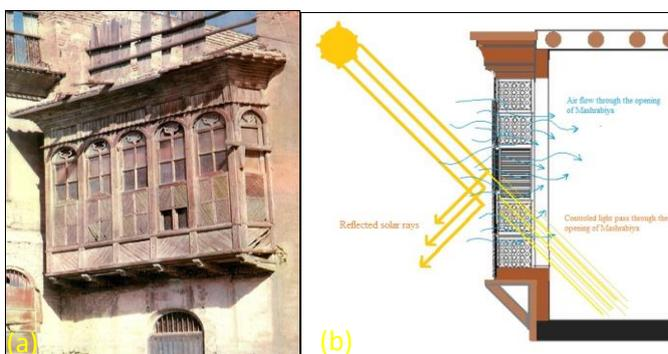
**Figure 2.** (a) Traditional wooden Mashrabiya located on the upper floor of Iraqi traditional house. (b) Section showing airflow through openings and shading of solar by Mashrabiya
