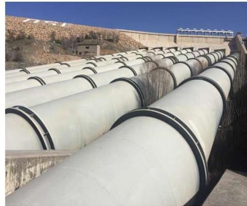
**Figure 1.** Penstock pipes
